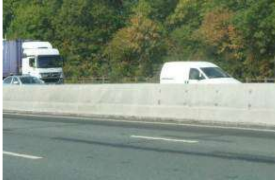
Figure 89 Rigid concrete barrier
