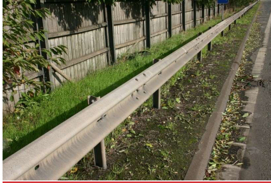
Figure 1 Steel Safety Barrier: Tensioned Corrugated Beam
