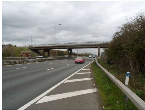
Figure 10 Steel Safety Barrier: Open Box Beam
