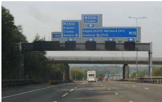
Figure 10 Typical portal gantry (two legs)
