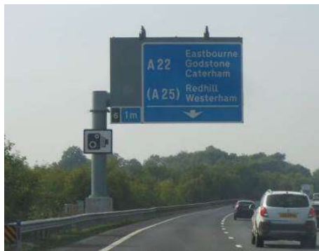
Figure 8 Typical sign-only cantilever gantry (one leg)
