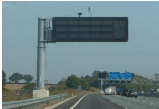
Figure 6 A cantilever gantry solely supporting an MS3 over lane 1
