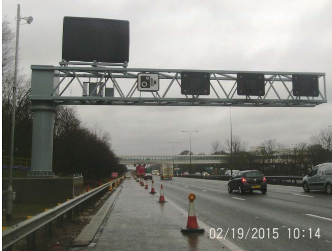
Figure 9 Typical super cantilever gantry
